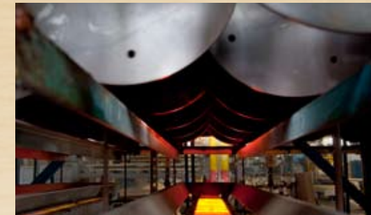
heat unit below cleaning line
